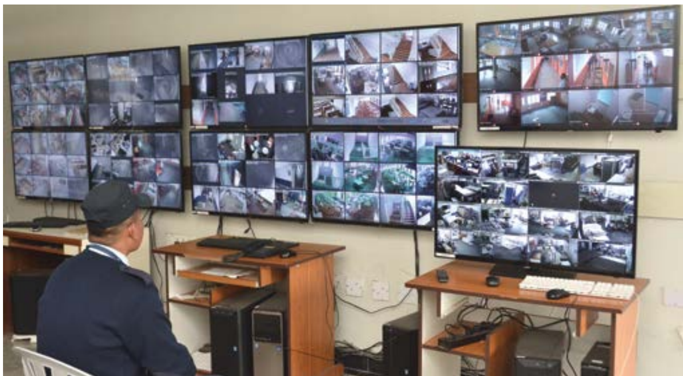
Security guard watching CCTV screens
