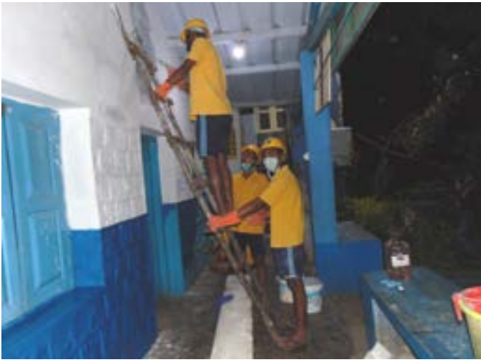
Students painting the walls of the local hospital in Kolikarai
